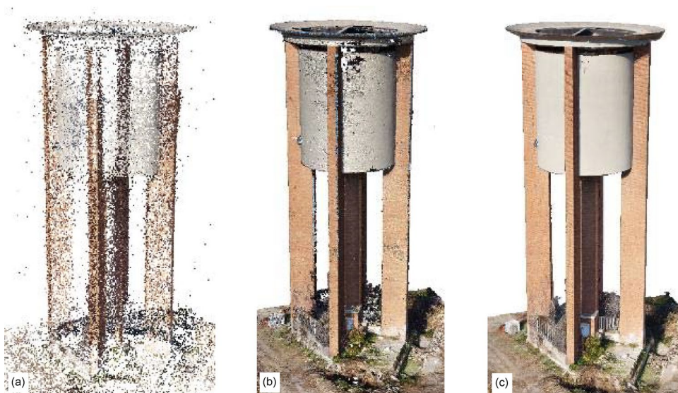
Fig. 3 Photogrammetric model of Tiburtina elevated water tank: sparse (a) and dense (b) point clouds, and 3D textured model (c)
